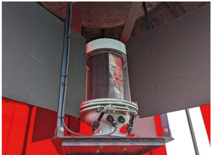
▲ The existing rotating optic
