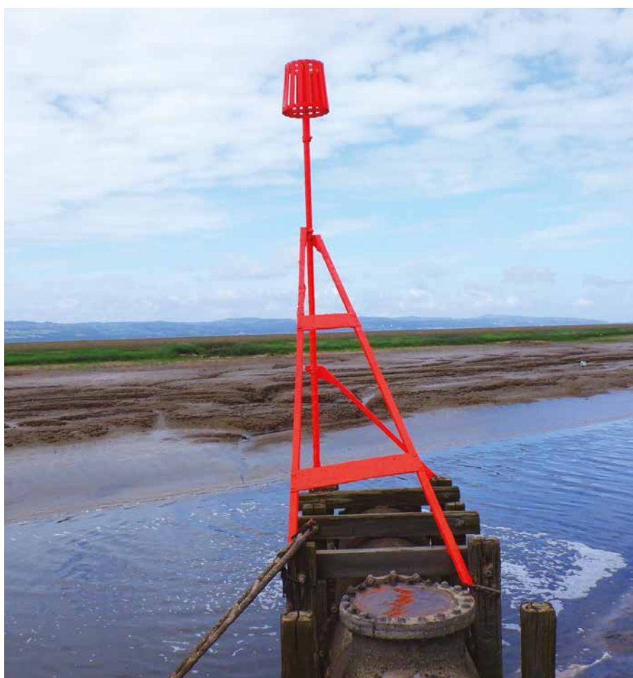
Above: Dwr Cymru Welsh Water beacon following maintenance.
