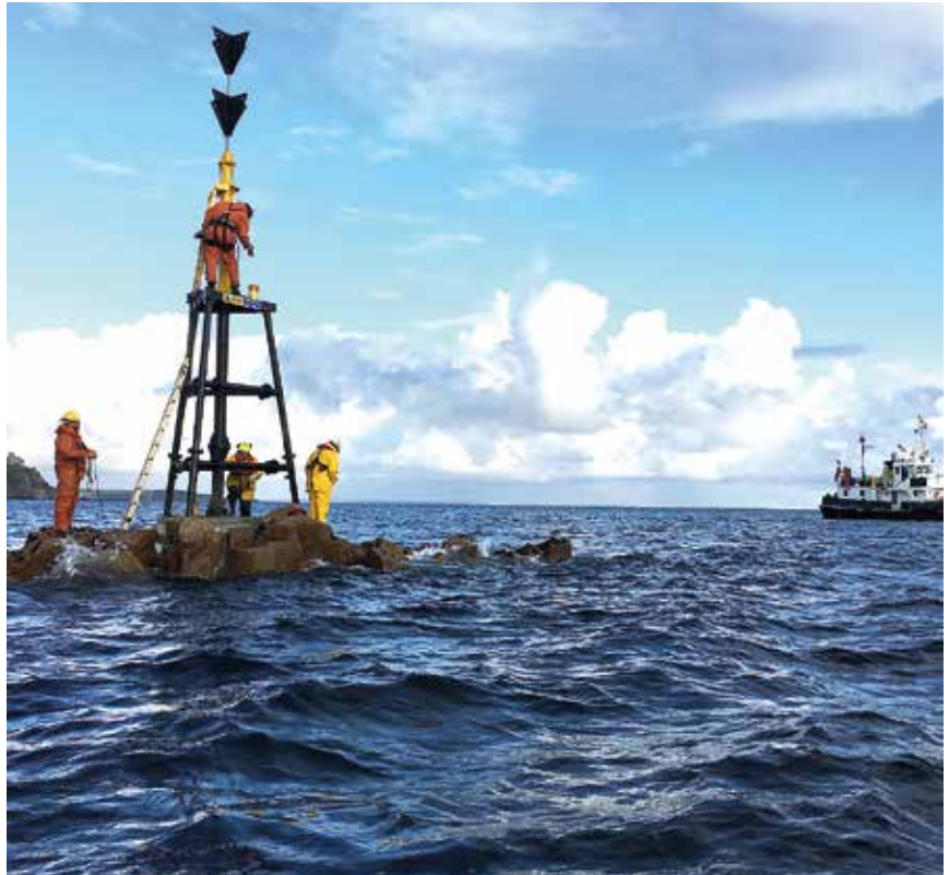
Installation team applying finishing touches
