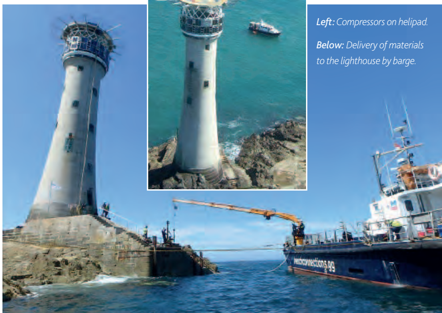
Rope access drilling.
