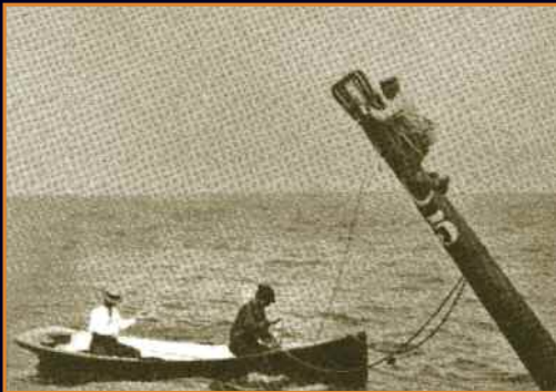
Above: Servicing underway on one of the Gedney Channel, New York harbour buoys. Possibly one of the first photographs showing a buoy being serviced on station.
